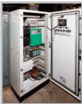
Cortina Rectifier Controls
